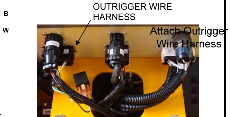
Figure 4-16. Bottom Side of the Ground (lower) Control Box.
