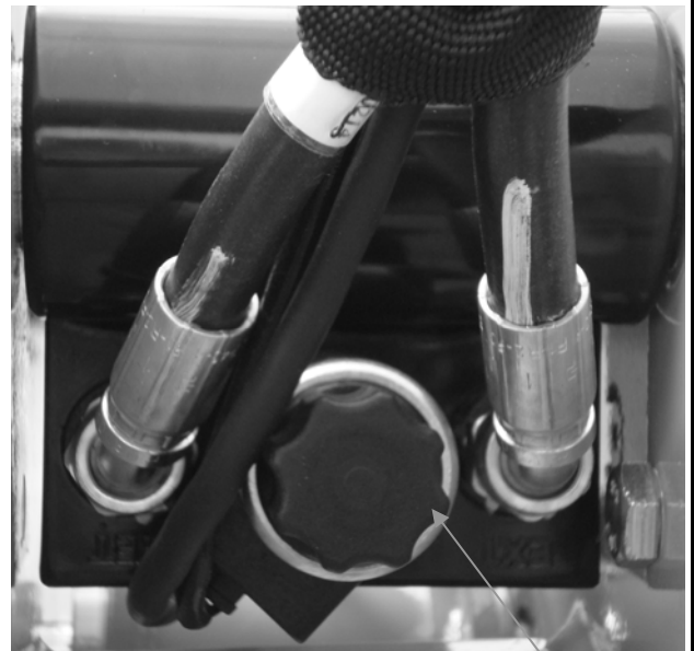
Figure 5-7. Cylinder Valve Removal
